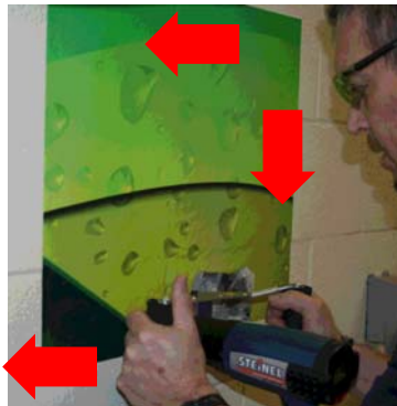
FIGURE 28 Lightly Set 3 Film Edges
