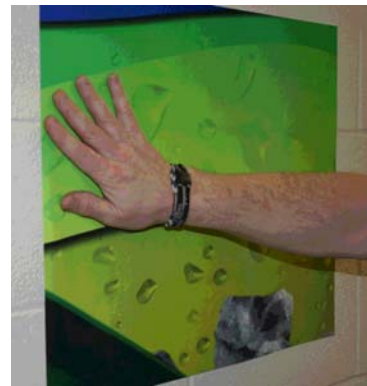
FIGURE 27 Use Your Hand to Pre-Adhere Film to the Wall
